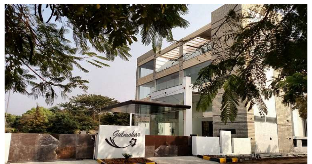
Club house at JR Greenpark
