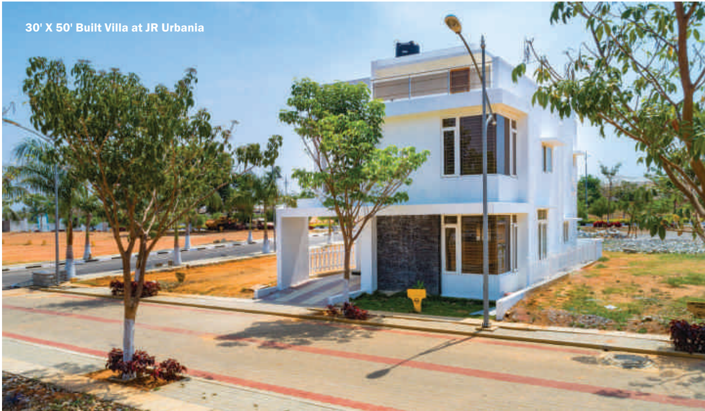
Built Villas at Villa street
